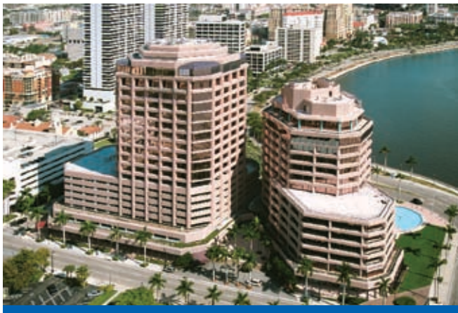
Phillips Point Office Buildings West Palm Beach, Florida
