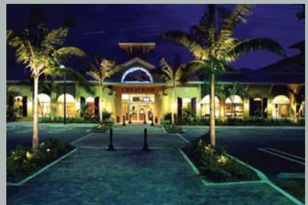
Creations of Pineapple Grove – This striking, 40,000-square-foot retail center included more than 6,000 linear feet of detailed wood crown molding installed on 186 display walls to conceal a wire raceway to service the data and video systems covering 30,000 square feet of retail space. For the 10,000-square-foot, Class A corporate offices, unusual forms and finishes were used to create a sophisticated, rich work environment.
