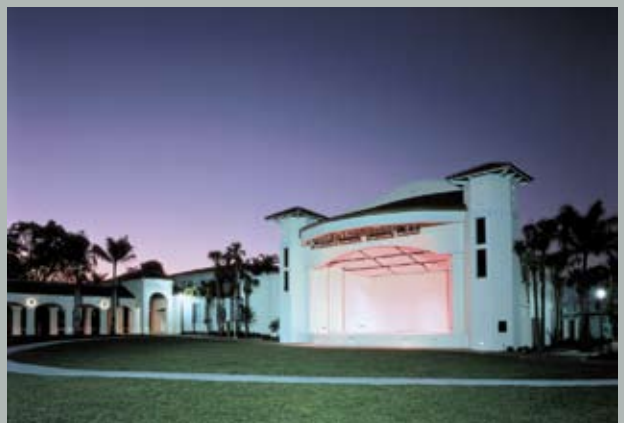
Old School Square Entertainment Pavilion – A state-of-the-art, outdoor performance stage, workshop, covered loggia and restroom/concession building was constructed on the Old School Square grounds.
