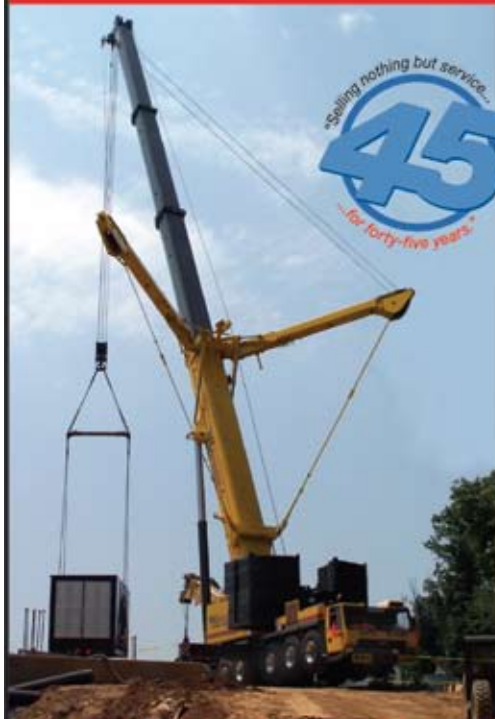
Grove 7550 All-Terrain Crane with Mega Wing Lift
