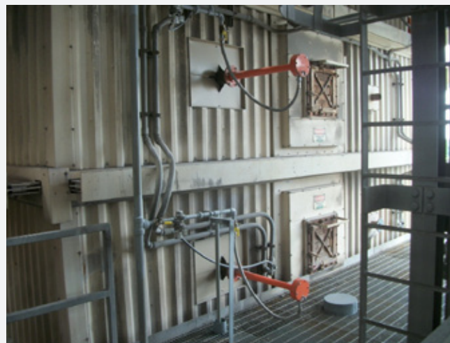
Sonic horn 010: The MARTIN® Sonic Horn is an acoustic cleaner that reduces system downtime, maintenance, and operating costs, while improving performance.
