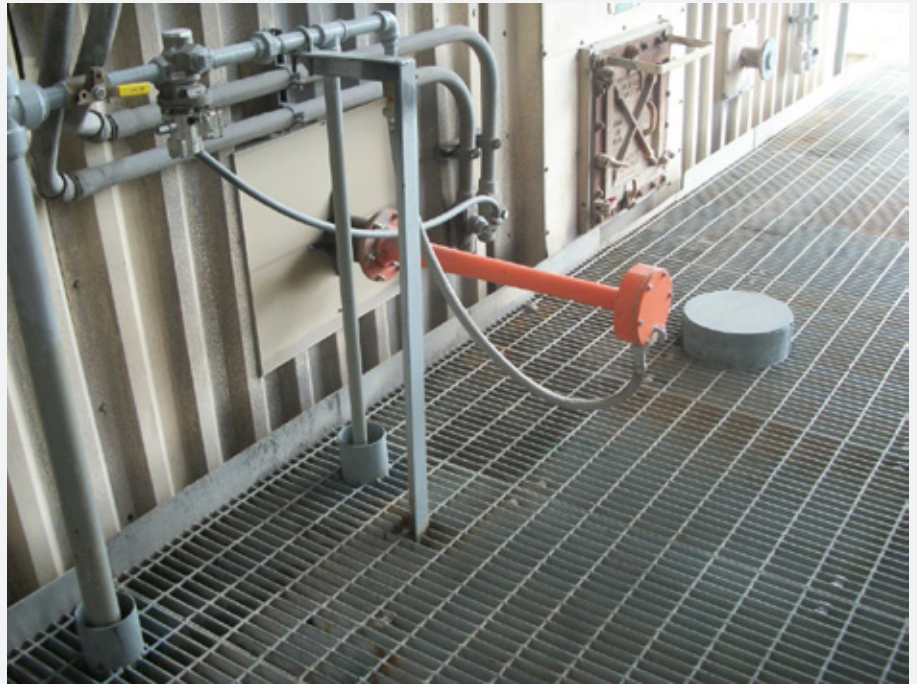
The new sonic horns are especially effective around pipes and behind obstacles, sonic energy de-bonds particulates with a 360-degree sweep, cleaning inaccessible parts.
