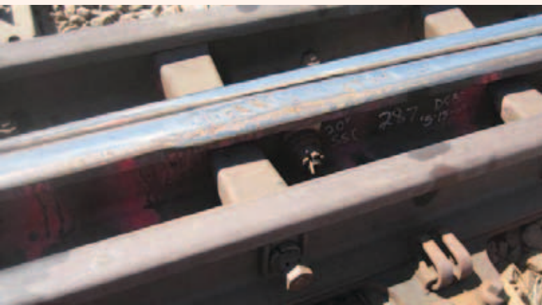
Figure 5. Conditions that could have been prevented with a switch grinding program.
