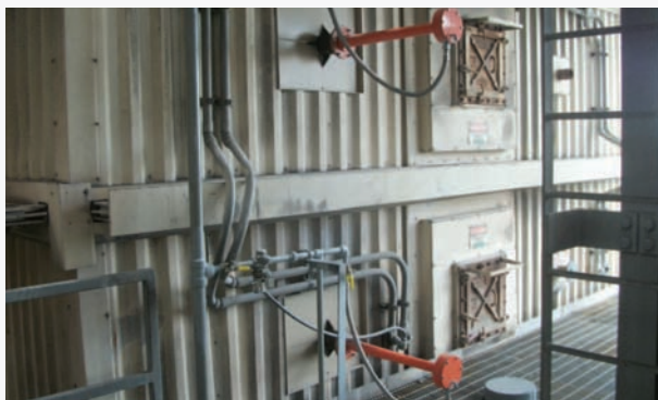
Sonic Horns comply with OSHA dB regulations for vessel interiors
