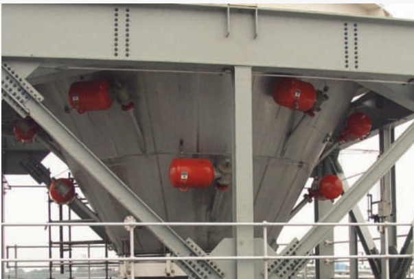
Air Cannons increase efficiency and productivity by improving material flow.
