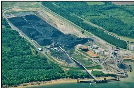
CCT is one of the largest rail to barge storage and blending facilities on the inland river system.
